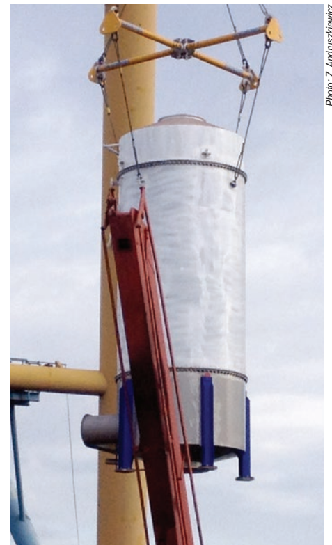
In the installation of scrubbers the shipyard - owned sheerleg REM 220 floating crane of 200 t lifting capacity was utilized.
